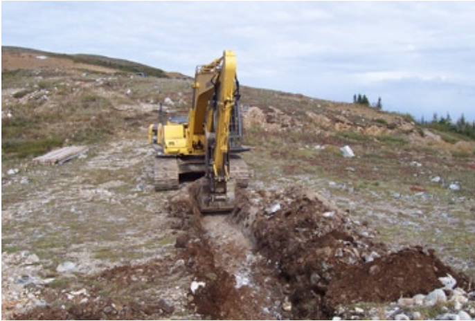
Trenching (photo courtesy of Mineral Resources Branch)
